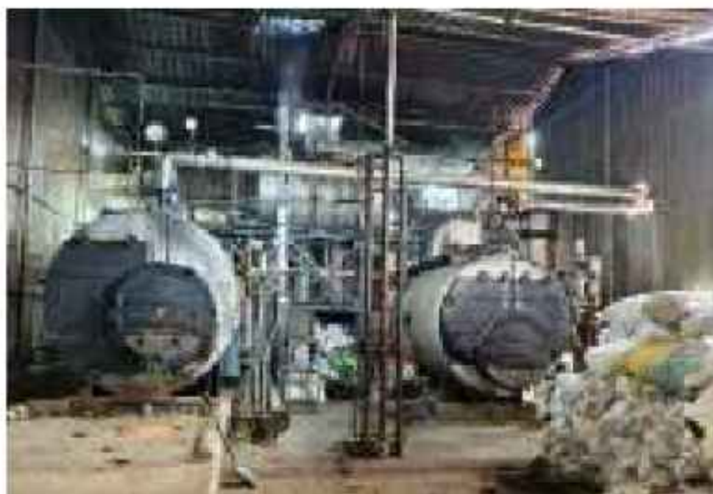
Fig. 27: Boiler
