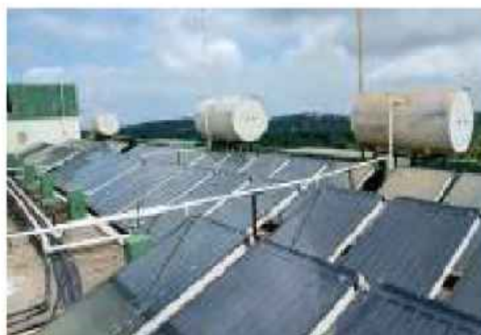
Fig 6: Solar panels for generation of hot water
