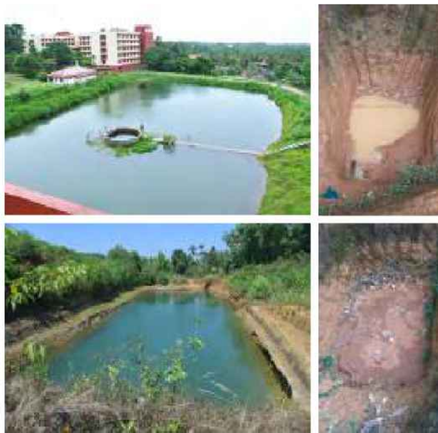
Fig.13: Rain water harvesting pond and percolation trenches
